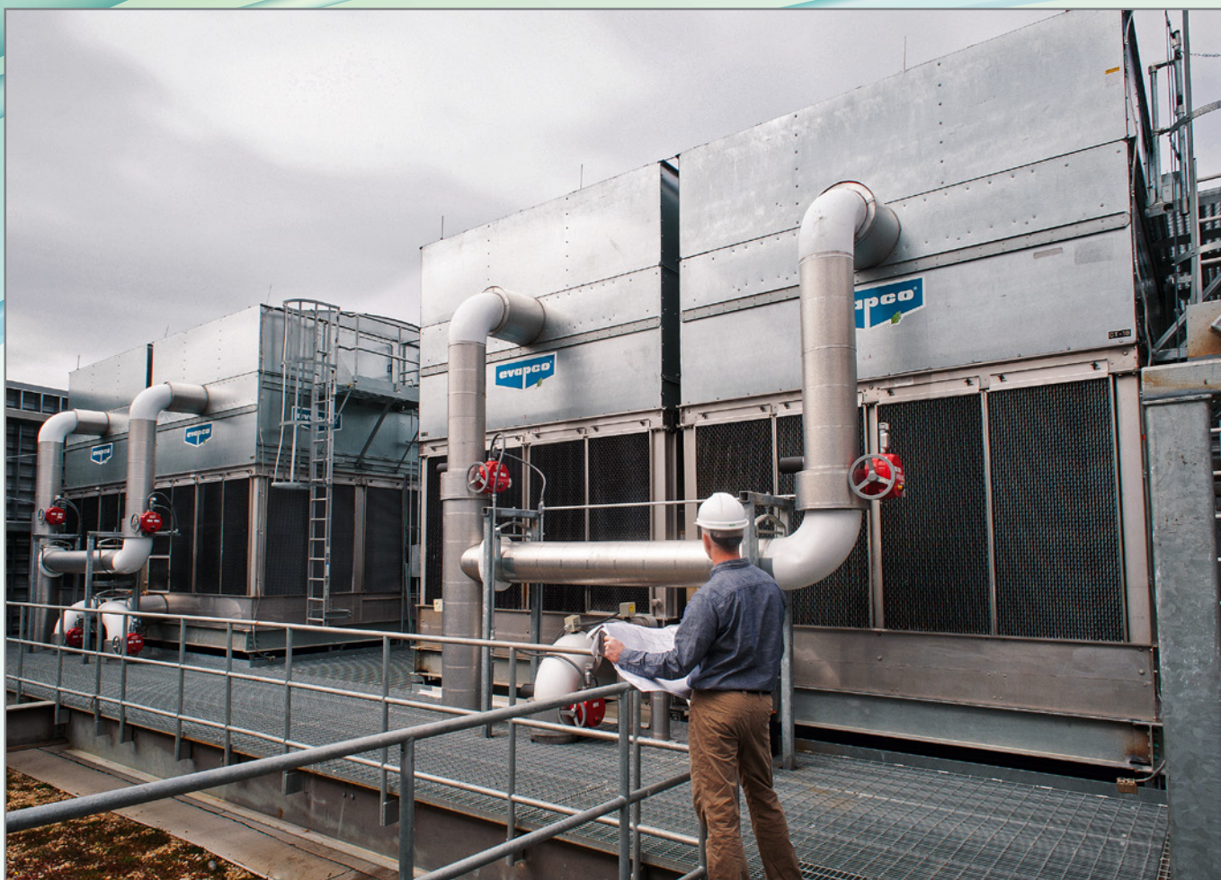
AT Cooling Tower with optional stainless steel basin.
