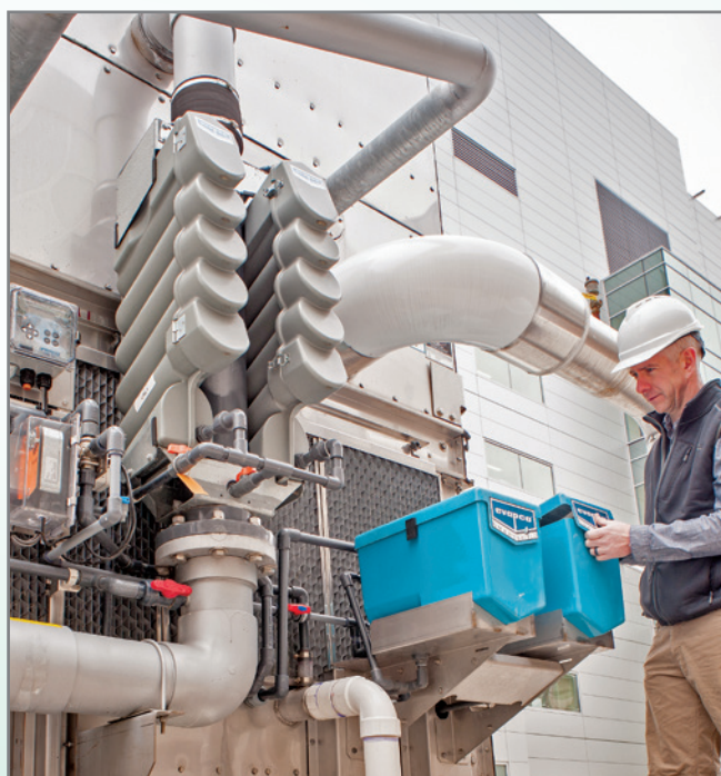
Smart Shield® Factory-Mounted Water Treatment System
