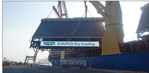
250-ton double fan module transportation
