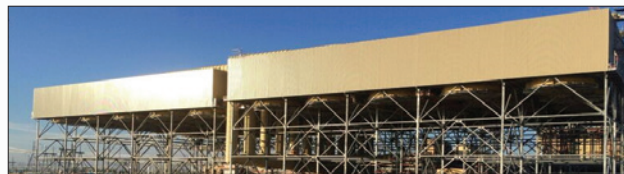
Butterfly arrangement to reduce overall height
