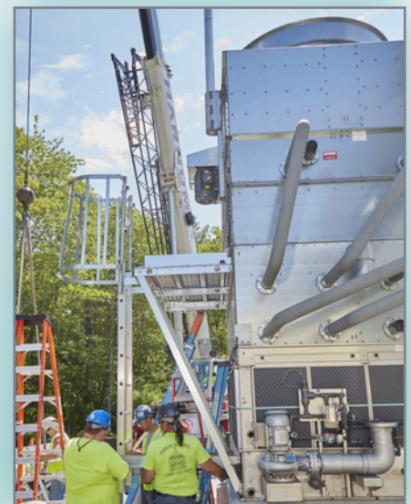
eco-ATWB-H Closed Circuit Cooler installation
